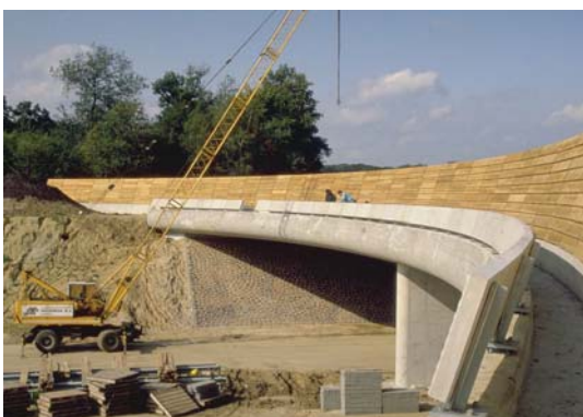
Green bridge construction in the Netherlands
